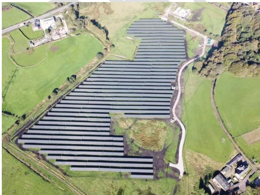
Fig. 7 Rochdale Council's 5.5MW Chamber House Solar Farm will provide enough electricity that could power 2,000 homes.
